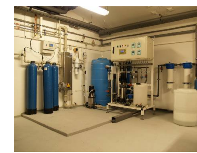
Production of DI water: resistivity 18 MΩ·cm @ 25 °C
